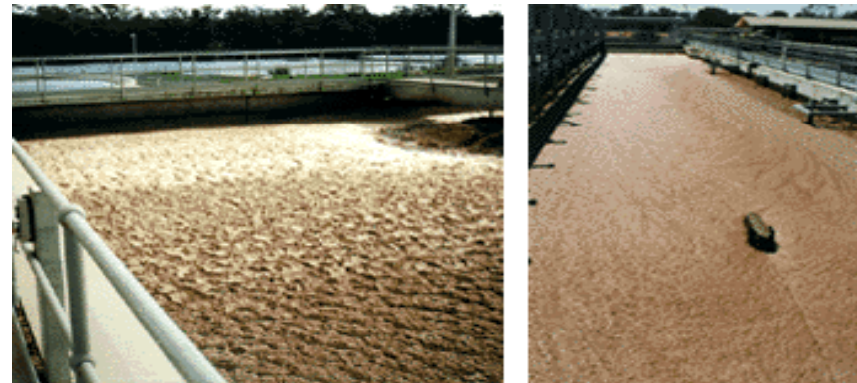
Figure 1. Foaming in two Australian activated sludge plants. Plant on right is an oxidation ditch with foam covering the dividing wall.
