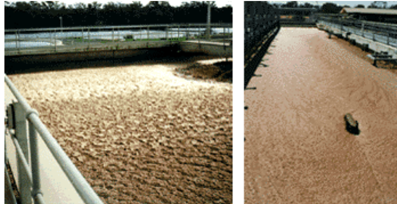
Figure 1. Foaming in two Australian activated sludge plants. Plant on right is an oxidation ditch with foam covering the dividing wall.
